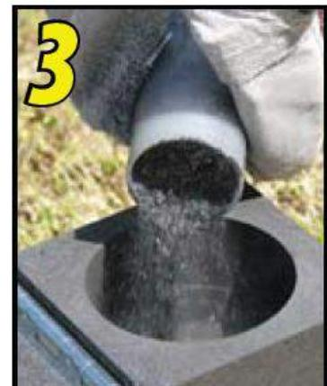
Pour exothermic welding powder in mold case.
