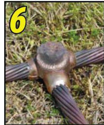
After having finished welding, cool the joint by normal air and then open the mold.
