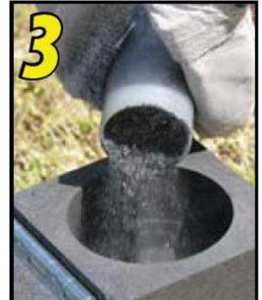
Pour exothermic welding powder in mold case.
