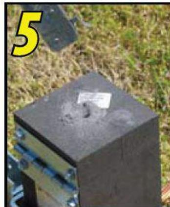
Ignite starter powder by flint igniter. Igniting reaction will occur by touch between spark and starter powder
