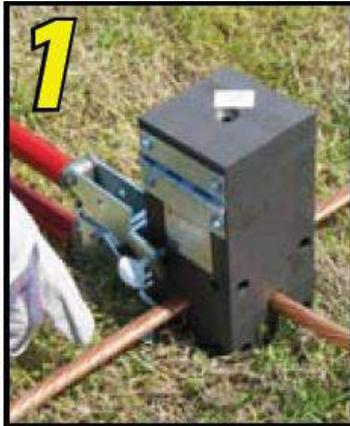
After preparing surface, install the mold-fixing handle, place the wire, and press it tightly.
