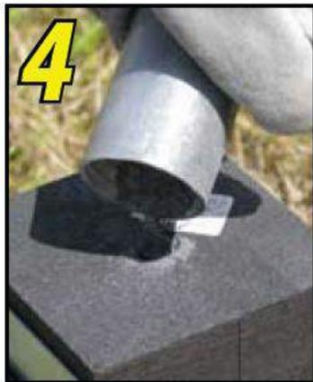
Pour starter powder contained at terminal of the tube on the exothermic welding powder .
