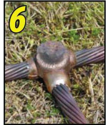
After having finished welding, cool the joint by normal air and then open the mold.
