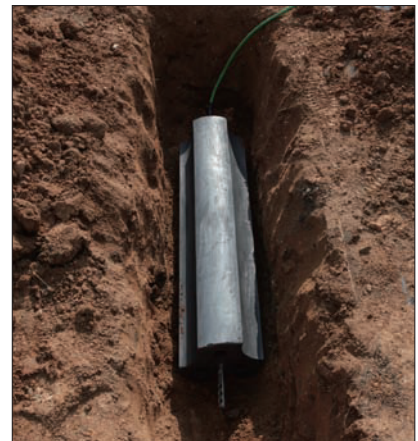
Place the Carbon Ground Module
