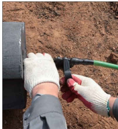
Put the insulating tape on the connecting part
