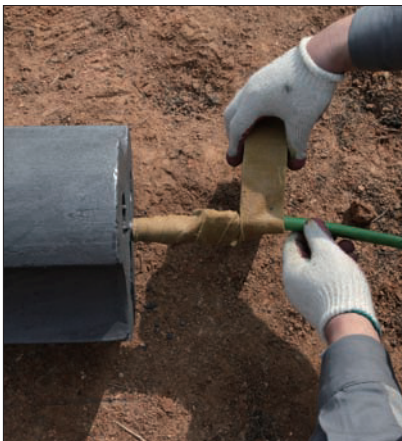
Put the rubber tape on the connecting part
